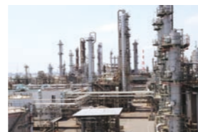
Yokkaichi Plant in Mie Prefecture where the plant tour was held
