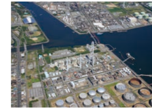
Panoramic view of Yokkaichi Plant
