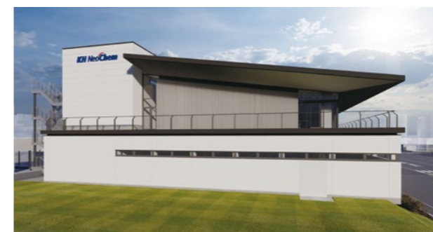
Building for quality control in Yokkaichi Plant, completion image
